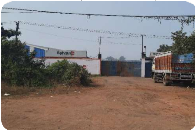
Main Gate (Entrance from NH-2)
