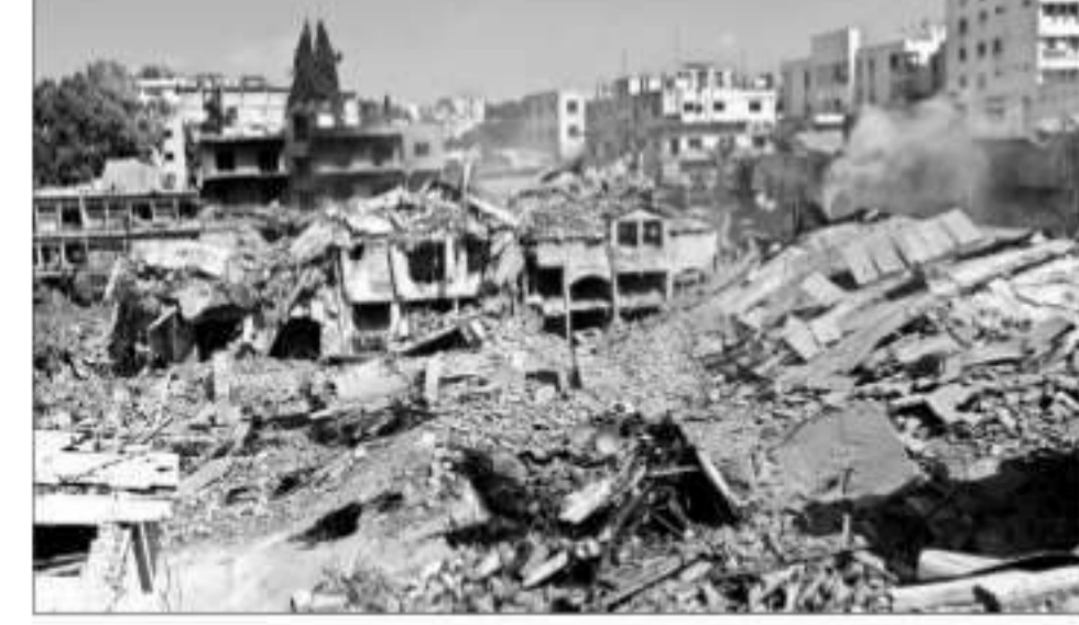
Damaged buildings in the aftermath of what security sources said was an Israeli strike on a commercial market in Nabatieh, southern Lebanon, on Sunday
