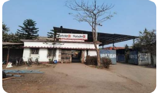
Main Gate (Entrance to Factory)
