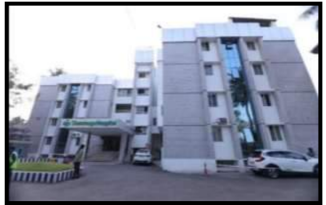
Hospital Main Block
