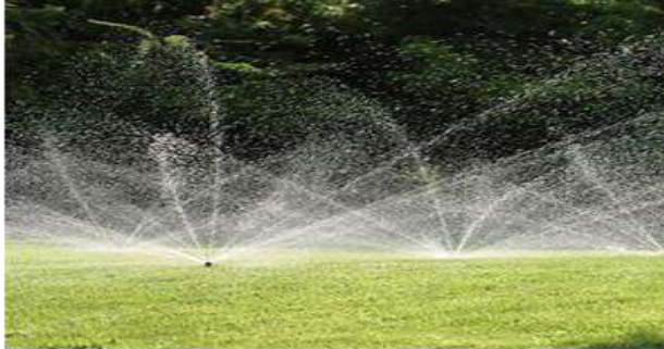
Landscape Irrigation System
