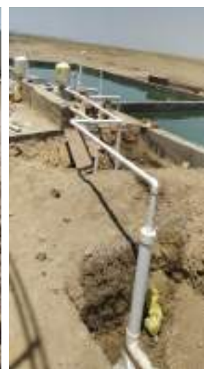
Pumping System Installation
