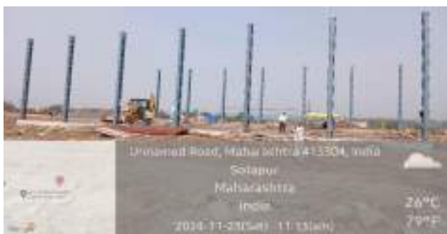
Mechanical Work at CBG Plant
