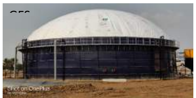
GFS Digester Tank (Completed)
