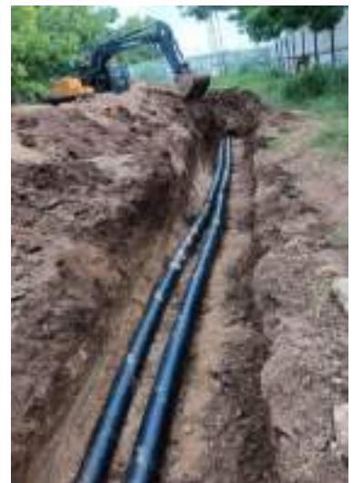
Laying of Pipe
