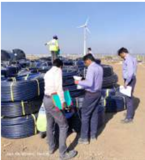
Supply of HDPE Pipe and Inspection at Site
