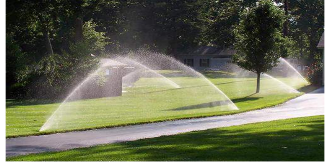
Sprinklers in Operation
