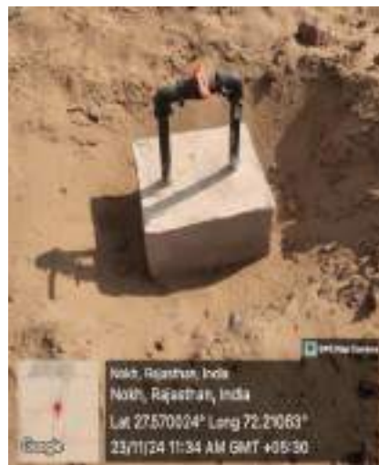
Installation of Fittings
