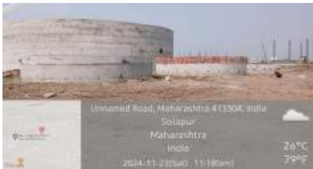
Outer View of CBG Plant
