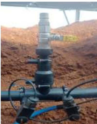
Electrofusion Jointing
