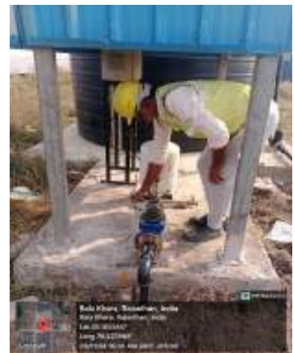
Testing of Pipeline with water
