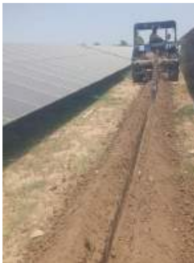
Excavation of Trench
