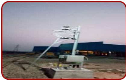
Ladder Assembly with DCS Mast Platform
