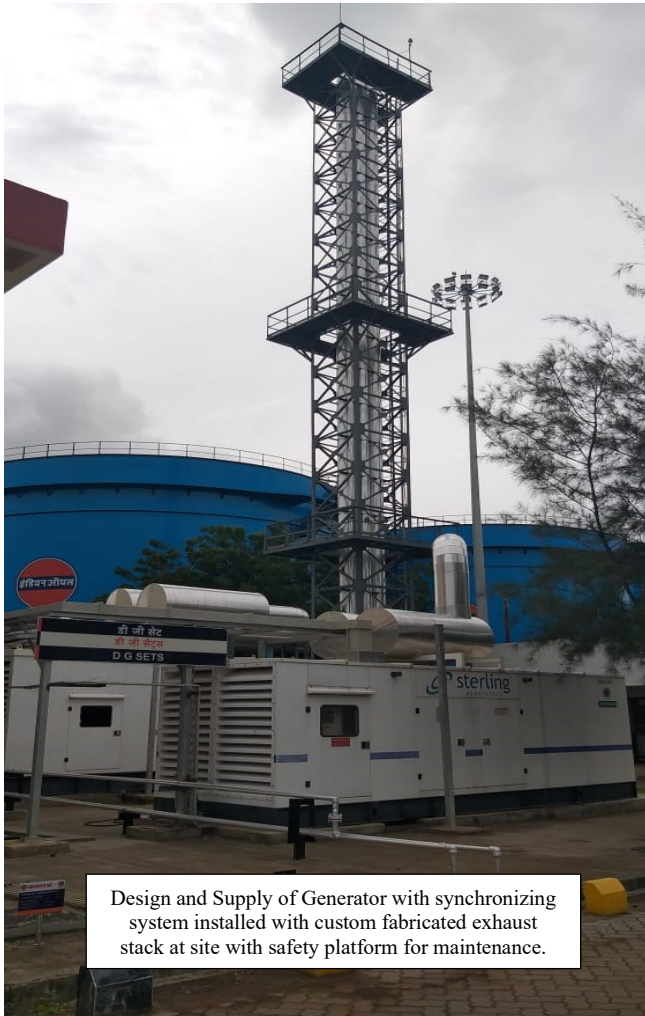
Generator with Exhaust Stack
